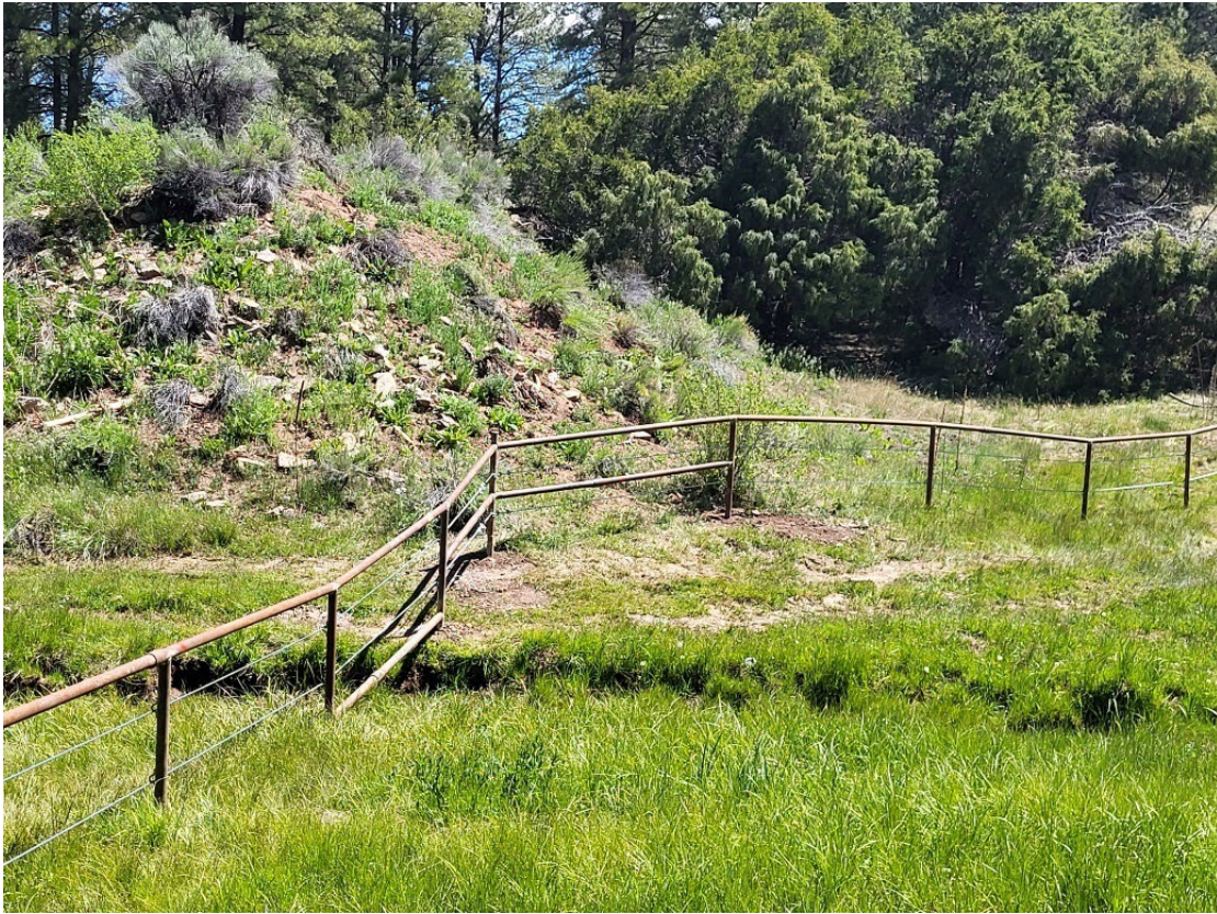
Figure 4. Pipe rail fence constructed at the headwaters of Bluewater Creek
